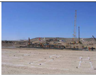
Figure 9 - Traçage des barrettes
