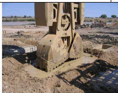
Figure 12 - installation de la machine de forage
