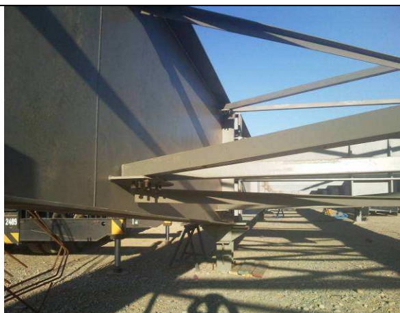
Figure 42- Contreventement horizontal anti-déversement
