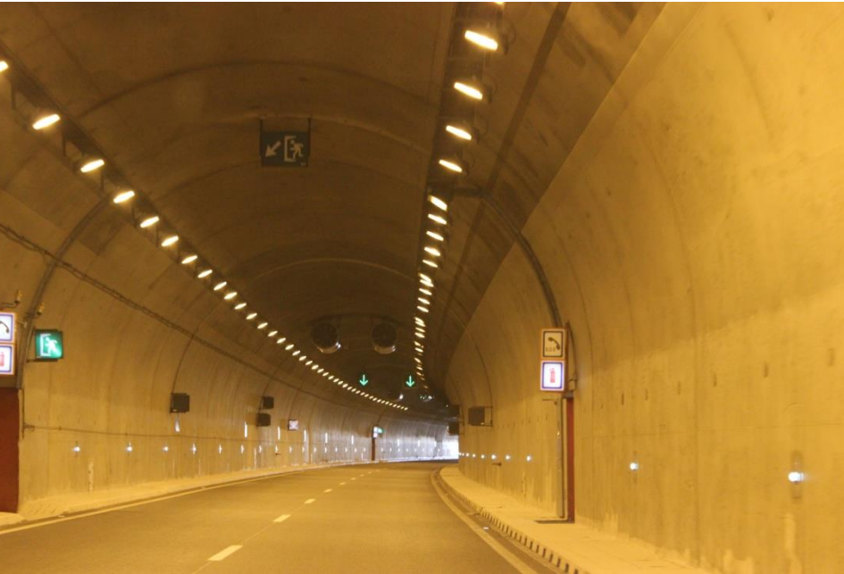
1 er tunnel autoroutier Autoroute Marrakech Agadir
